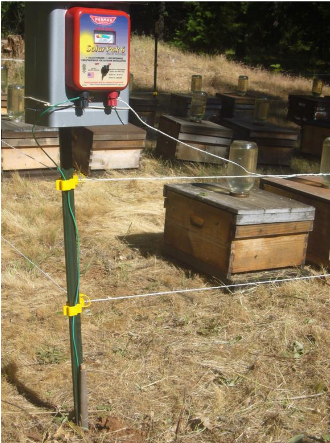
Solar charger, ground wire protected from weed whacker and then run shallowly underground to the ground rod (not shown). Note detail of how I attach the hot jumper—I unwind a bit of the hot wire and weave the jumper into it.
