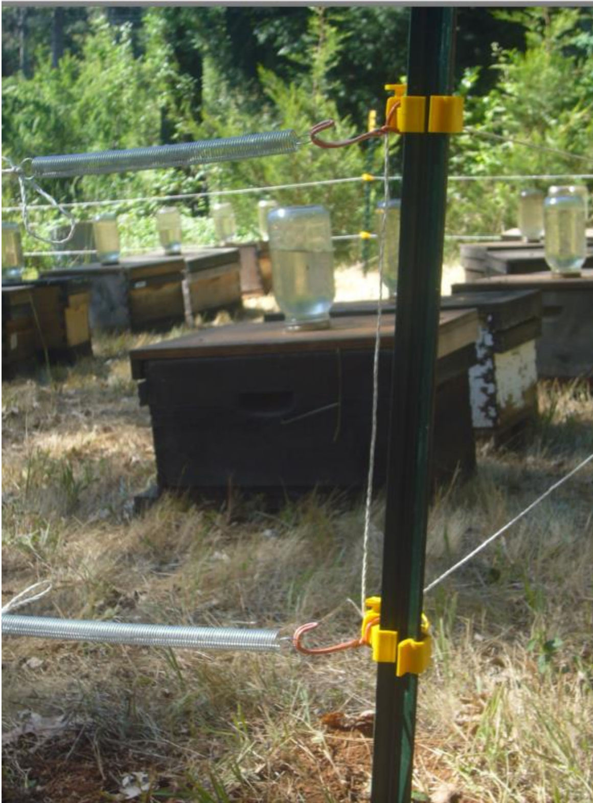
Corner detail. The orange 12-ga hook is twisted to the insulator, and must not contact the fencepost.
